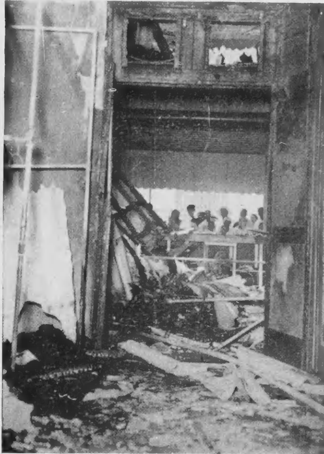
Fire damage to the interior of the Band Box Dry Cleaners in San Nicolas is shown by this picture taken from the courtyard in the rear of the building. Places damaged or destroyed by the February 10 fire were the Band Box, Abma's Store, Aruba Trading Annex, El Liberator, Aruba House of Art, De Vries' Bar, Maritime Bar, and the Target Bar.
